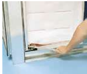
The fitting of the air filter with parallelogram towards the gasket ensure airtightness
